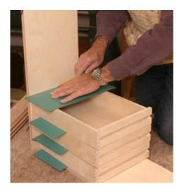
**Align the drawers.** Before hanging the drawers, use the drawer boxes and some laminate shims to mark the location of the bottom shelf (part of the gallery). Stack the drawers with laminate shims to mark the location of the dado in the cabinet side.
